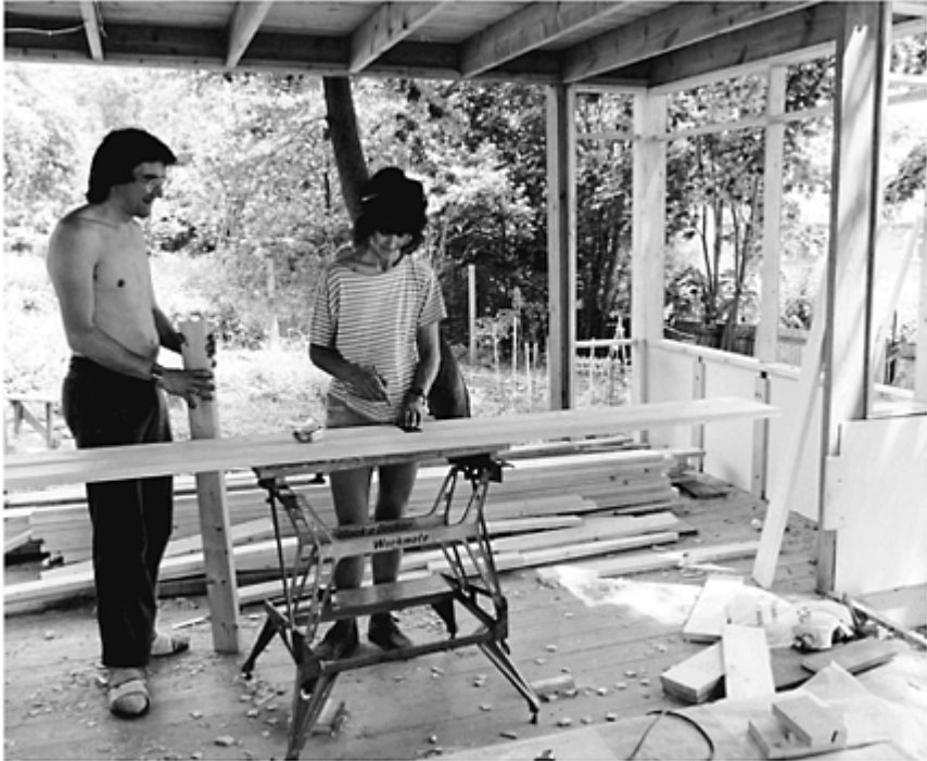
04.03 –Lewisham self-builders at work in a half-constructed Segal House.
