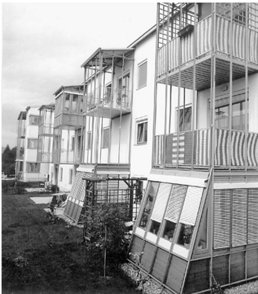
09.14 –Housing at Graz-Ragnitz, view of garden side, showing the varying use of the projected balcony.
