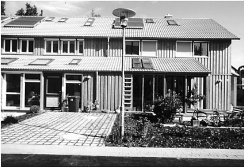
10.14 – Ecological houses in Edenkoben.
