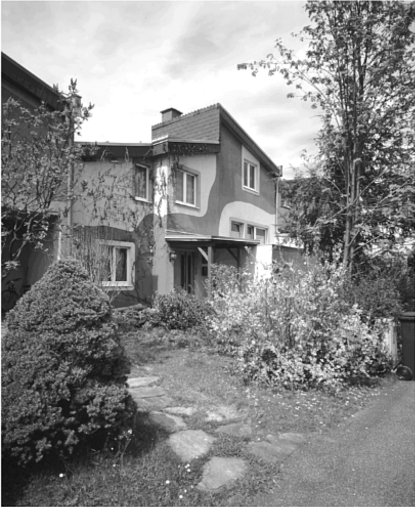
08.09 – Typical houses at the Eschensiedlung Deutschlandsberg, Styria (south of Graz) 1972 onward. Architect Eilfried Huth did his best to allow each family to develop their house according to their own needs and preferences, and no two have the same floor plan.
