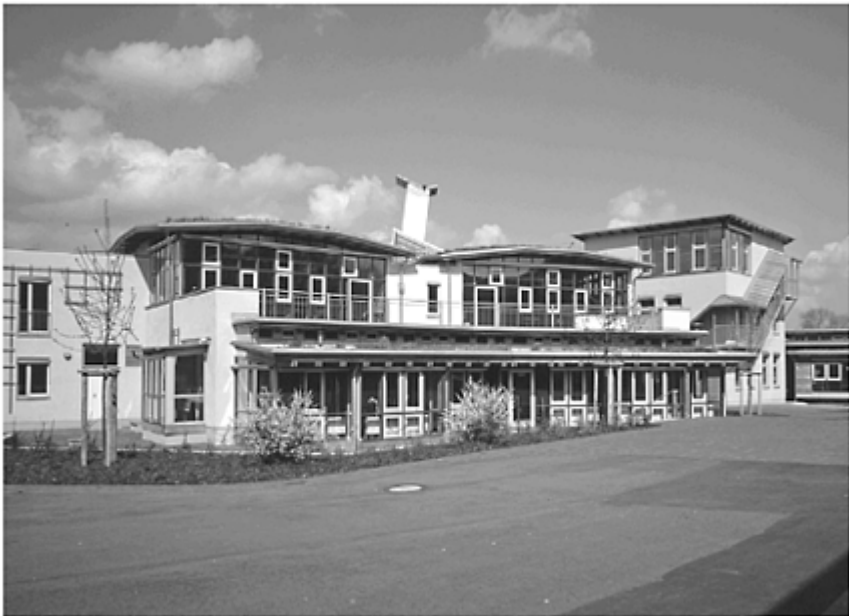
12.01 –Gelsenkirchen school from the front. The school cafeteria on the ground floor with classrooms above, and administration on the right; behind is the ventilation stack for the theatre.
