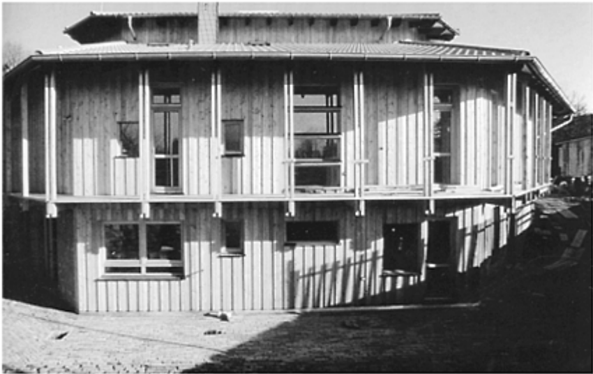
10.11 – Landau cultural centre, a self-build project by the Landau youth choir designed by Peter Sulzer 1985-7. The hall for concerts and rehearsals is surrounded by offices and dwellings.
